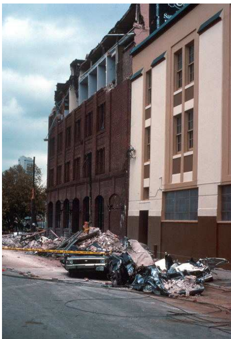
Cars crushed by falling masonry, which killed 5 people leaving work. Loma Prieta earthquake, 17 th Oct. 1989. (From the US Geological Survey Photographic Library at: http://libraryphoto.cr.usgs.gov Slide 1-1 USGS Open File Report 90-547)
