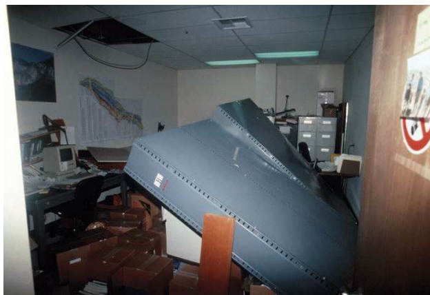
Unfastened bookcases in the headquarters of the US Geological Survey at Menlo Park, California, which fell during the Loma Prieta earthquake, 17 th October 1989 Slide VI-1. (From the US Geological Survey Photographic Library at: http://libraryphoto.cr.usgs.gov Slide VI-1 USGS Open File Report 90-547)
