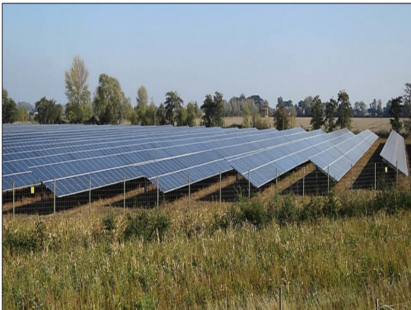
Mingay Farm solar farm, bank of the Great Ouse, near Aldreth, Cambridgeshire, England. Solar panels are angled to collect the most solar power from the Sun.
