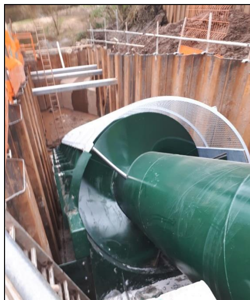
The River Dane Archimedes screw under construction (March 2021. Photo: Peter Lane)
