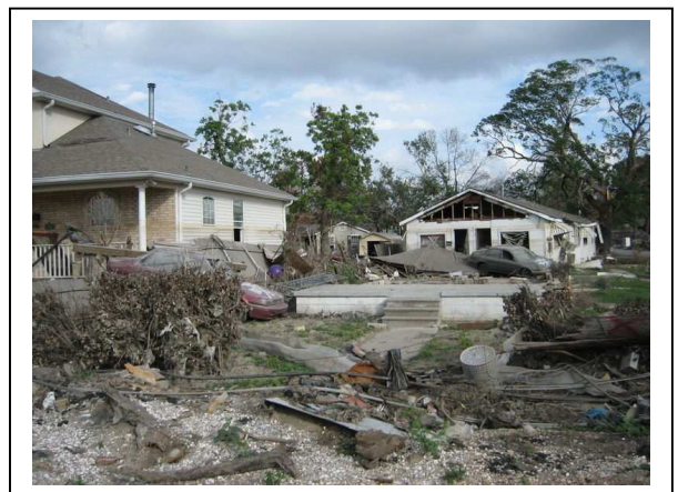
New Orleans after Hurricane Katrina: the flood damaged West End neighborhood, Bellaire Street, near the 17th Street Canal levee breach. Flood waters flung around automobiles, knocked a house off its foundation and moved it half a block away.
