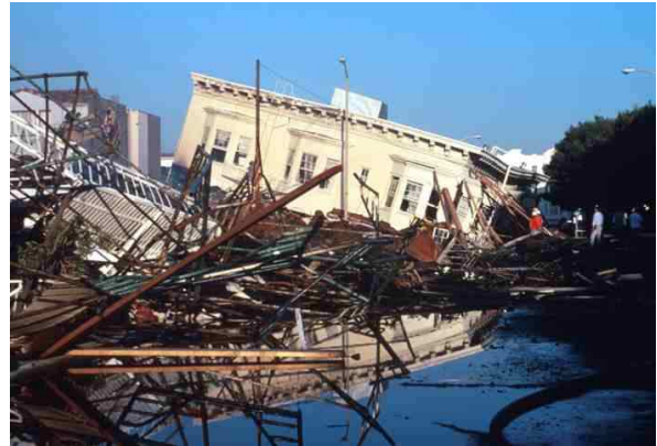
Collapsed and burned buildings in the Marina District, San Francisco. Loma Prieta, California, Earthquake October 17, 1989.
