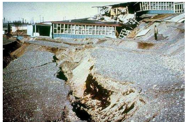
Government Hill Elementary School torn apart by subsidence that occurred during the 1964 earthquake. Notice the large crack in the foreground that also was caused by the earthquake, (9.2 magnitude).
