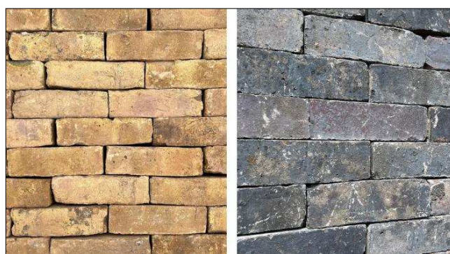
Fig 5. London bricks (left), Staffordshire Blue (right) from Reclaimed Brick Company
