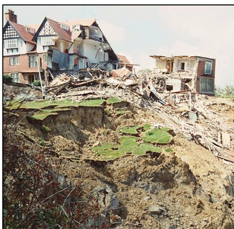
Holbeck Hall Hotel after the landslide (© BGS).
