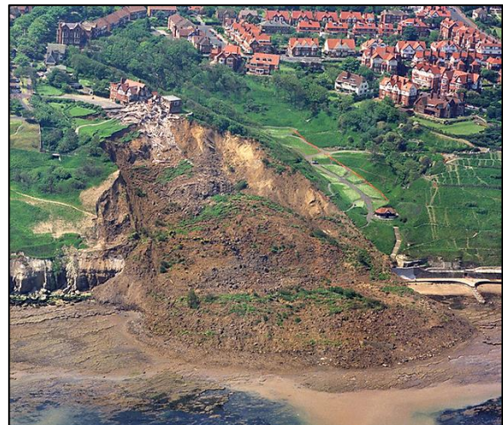
The Holbeck landslide. (© BGS).
