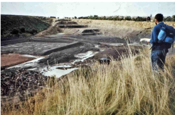
The clay pit being prepared to receive landfill
