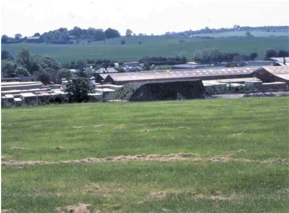
Stairfoot brickworks. The foreground is landfill in a former clay pit. The dark mound is a vast compost heap and finished bricks are stacked to the left of the picture.
