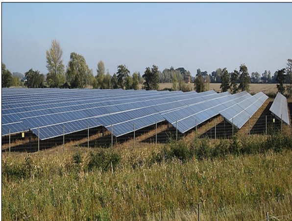
Mingay Farm solar farm, bank of the Great Ouse, near Aldreth, Cambridgeshire, England. Solar panels are angled to collect the most solar power from the Sun.
