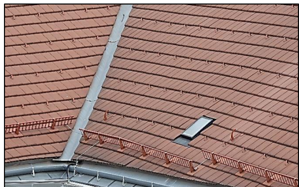
Snowguards on a roof in Vienna, Austria.
