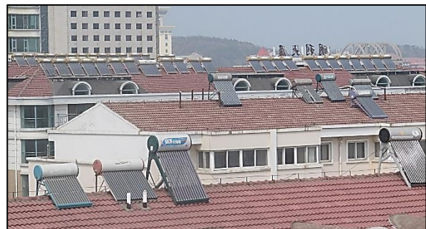
Solar hot water panels in Weihai, Shandong province, China.
