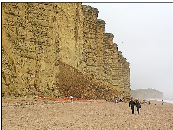
A recent cliff fall near Bridport on the south coast of the UK. (Peter Kennett).
