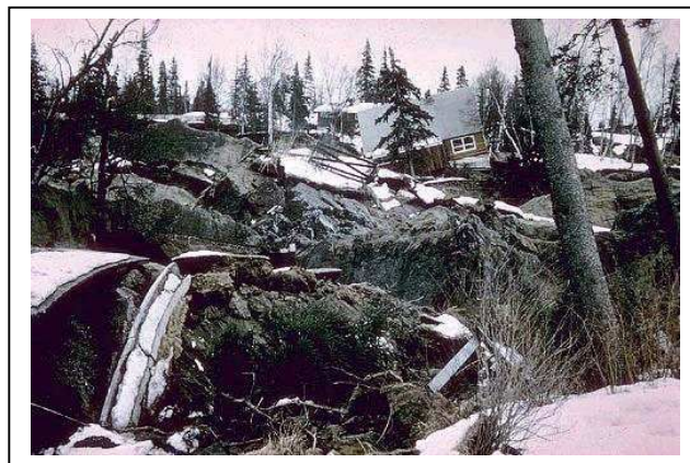
Buildings carried by a landslide - the Turnagain Heights landslide in Anchorage. 75 homes slumped, twisted, or collapsed when liquefaction of subsoils caused parts of the suburban area to move up to 700 metres during the 1964 earthquake (9.2 magnitude).
