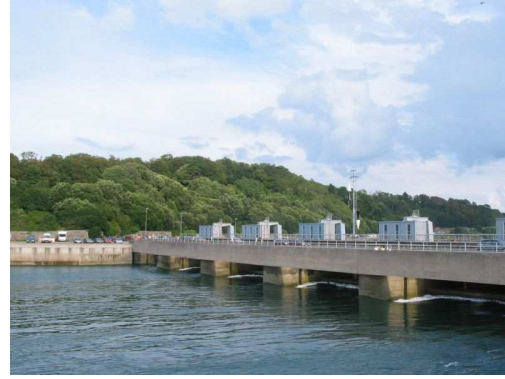
Dam of the tidal power plant on the estuary of the Rance River, Bretagne, France.
