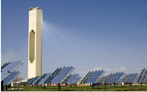
The first commercial solar power plant at Sanlúcar la Mayor in Spain.
