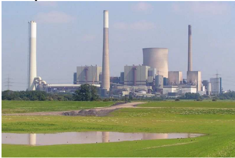
STEAG coal power plant, Rheinberg, Germany.
