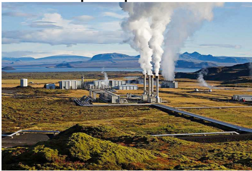
Nesjavellir Geothermal Power Plant in Iceland.
