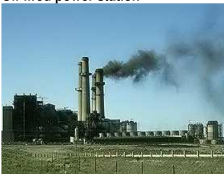
An oil power plant in Iraq.
