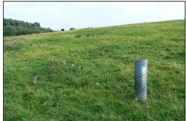
Vent to release potentially dangerous methane from landfill filling an old quarry, Severn Way, near Hempsted, Gloucestershire, UK.
