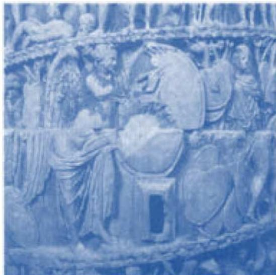
Figure 21 - A detail of the dislocation of two sections of the Marco Aurelio column
